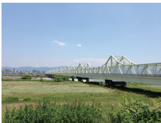
Fig. 1. (Color online) Bridge of study (Chosei Bridge).
