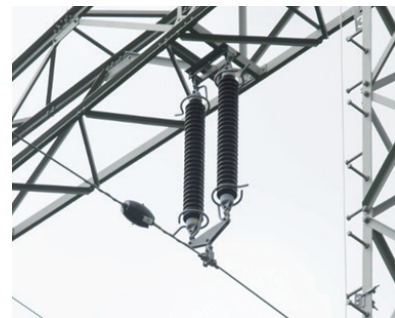
Fig. 7. Sensor node on a power line.
