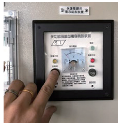
Fig. 14. (Color online) CTD discharge test.
