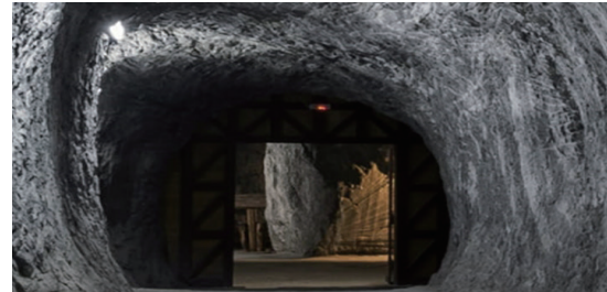
Fig. 9. (Color online) Tunnel construction site.
