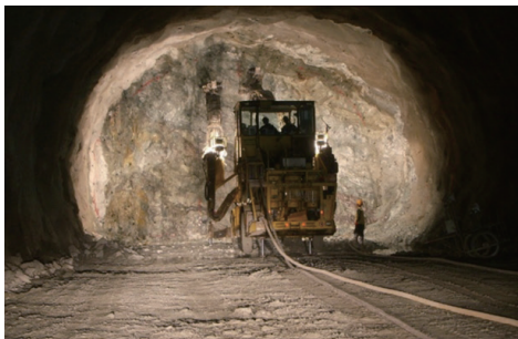
Fig. 3. (Color online) Tunnel excavation work.
