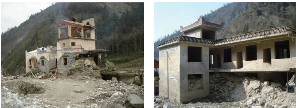
Fig. 2. (Color online) House destroyed by the debris flow along Longxi River Basin.
