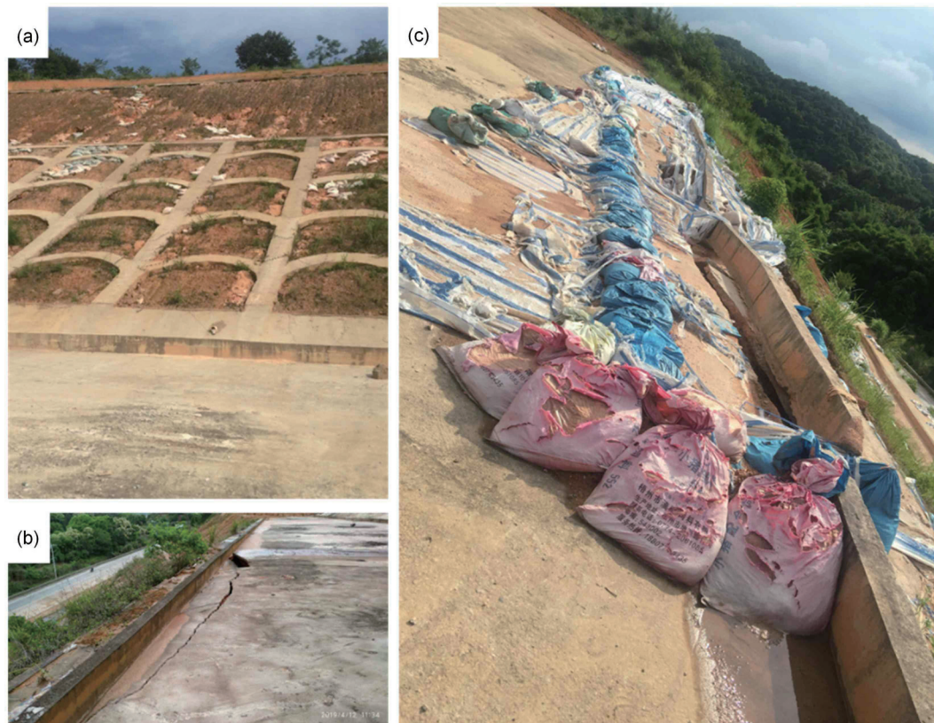
Fig. 11. (Color online) Photographs of field investigation. (a) Third-level slope. (b) Cracks on secondary berm. (c) Dislocation of the retaining wall top in the secondary berm.
