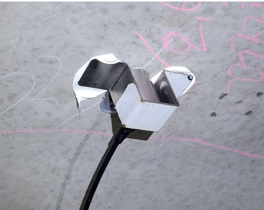
Fig. 23. (Color online) On-site installation of AE sensors.
