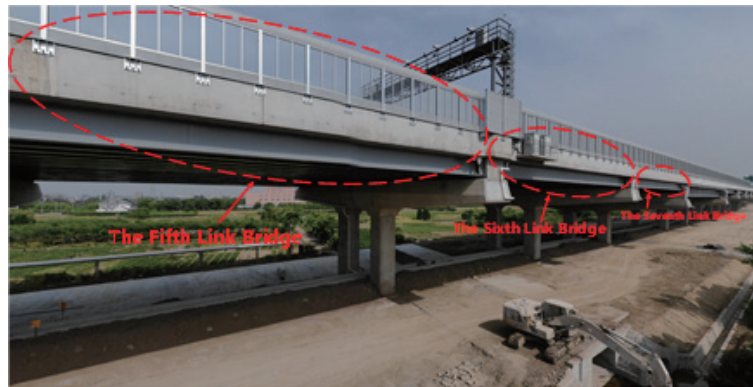
Fig. 23. (Color online) Photograph of an actual bridge.
