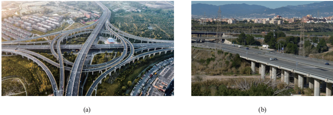
Fig. 1. (Color online) Clusters of prefabricated beam bridges. (a) Urban elevated viaduct cluster and (b) cluster of highway girder bridges.
