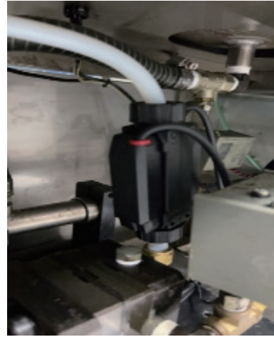
Fig. 8. (Color online) Curing agent pipeline.
