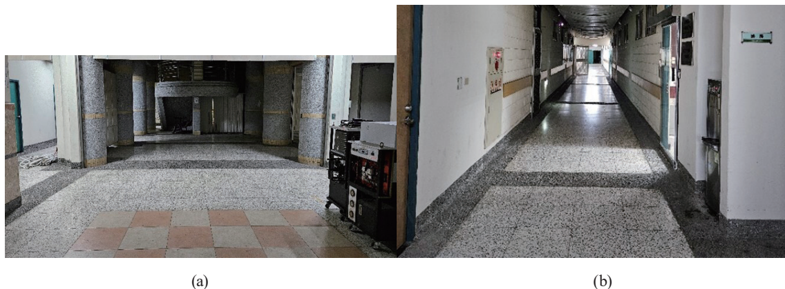
Fig. 11. (Color online) Images of the basement of the Engineering Building: (a) basement staircase and (b) basement hallway.
